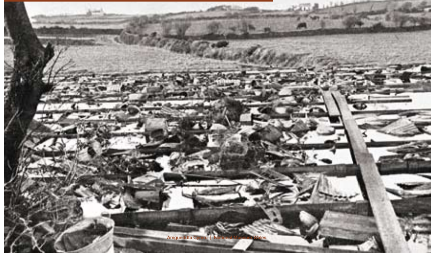
Adennill copr o byllau dyddodi Mwynglawdd Mona a Parys, Sir Fôn Copper salvage from precipitation pits, Mona and Parys Mine, Anglesey
